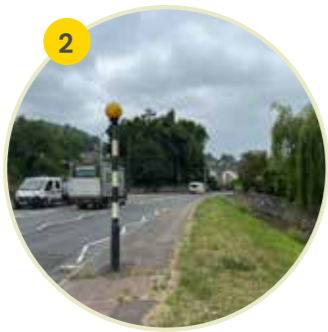
Poor quality environment around bus stop and school entrance
