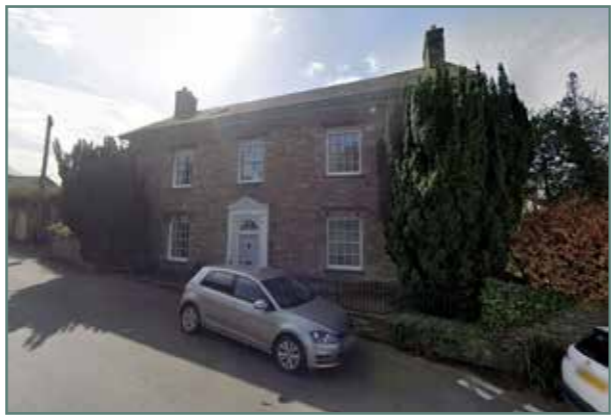
Traditional stone buildings
